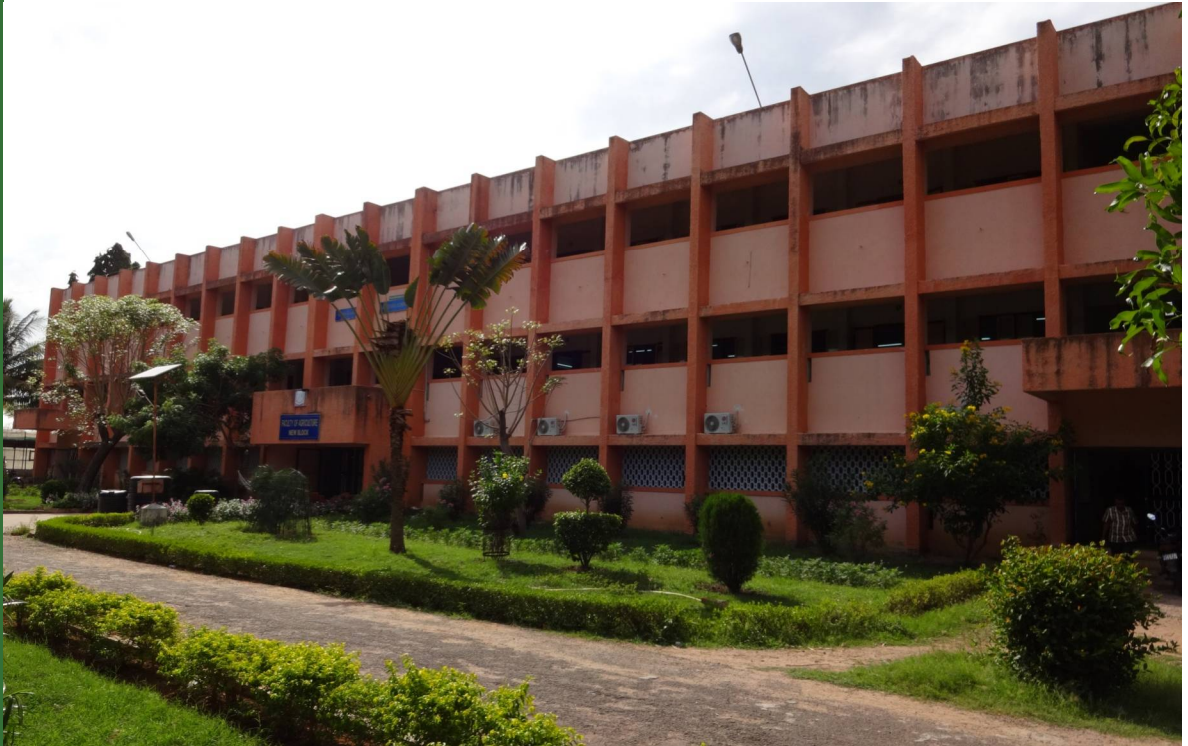
Class Rooms - New Block
