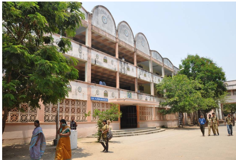
Class Rooms Platinum Jubilee Block
