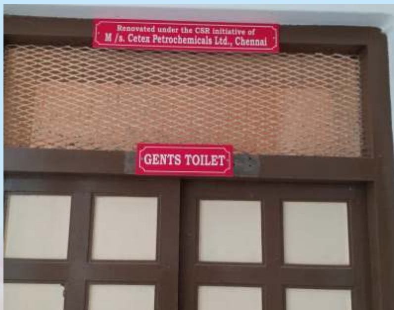
Renovation of toilet block at North West corner of FEAT building under the CSR Initiative of Cetex Petrochemicals Ltd., Chennai
