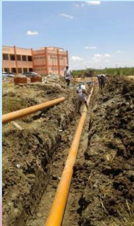
Re-drainage connection from Tech-Park to O.P drainage pumping station well
